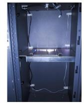
Figure 1. Ensure power and phone - cords are routed through cable clips.
