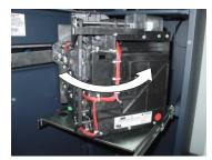
Figure 4-15. Rotate mechanism to operate position (counterclockwise).
